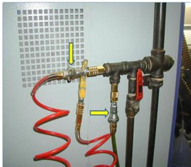
In line air reducers: Previously, all equipment was connected directly to the compressed air system at 120 psi – more pressure than many machines and tools needed. Devices were installed (see arrows) that limit air pressure to 60 psi or 90 psi. Estimated savings: 17,365 kWh or \$2,777.
